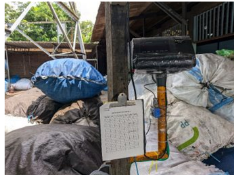
Facility located under 150 Kv High Voltage Electric Tower, which do not meet Horizontal Clearance Minimum standard required by Ministry of Energy and Mineral Resources Regulation No. 13 Year 2021
